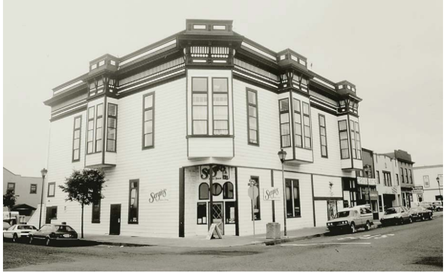
Figure 1.2e Bay windows are used to capture as much light as possible in a mild but very overcast climate such as that found in Eureka, California.
