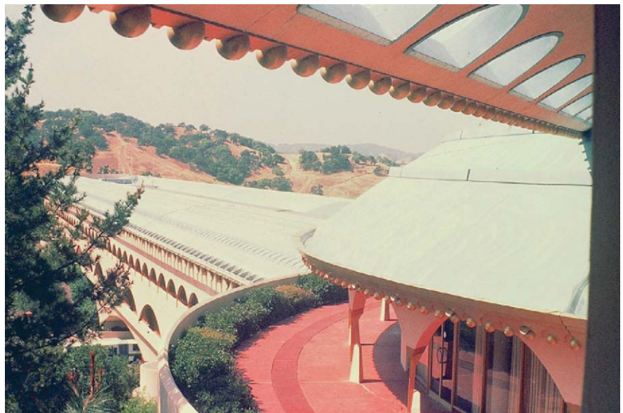
Figure 1.3f The exterior windows of the Marin County Civic Center are protected from direct sun by an arcade-like exterior corridor.
