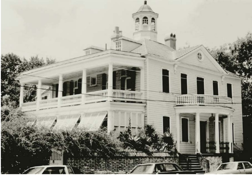
Figure 1.2b In hot and humid climates, natural ventilation from shaded windows is the key to thermal comfort. This Charleston, South Carolina, house uses covered porches and balconies to shade both windows and walls, as well as to create cool outdoor living spaces. The white color and roof monitor are also important in minimizing summer overheating.
