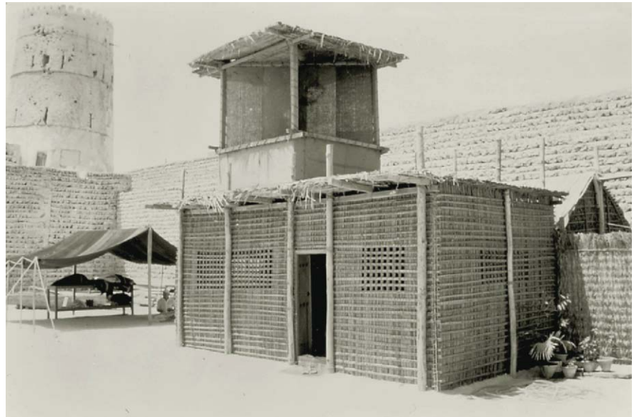
Figure 1.2d When additional ventilation is desired, wind scoops can be used, as on this reconstructed historical dwelling in Dubai. Also note the open weave of the walls to further increase natural ventilation. Although this is a desert area, lightweight construction is appropriate because the region along the Persian Gulf is humid. (Photograph by Richard Millman.)
