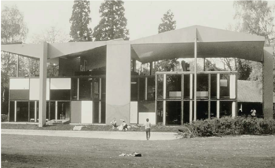
Figure 1.3g The Maison de l'Homme in Zurich, Switzerland, demonstrates the concept of the parasol roof. The building is now called Centre Le Corbusier. (Photograph by William Gwin.)
