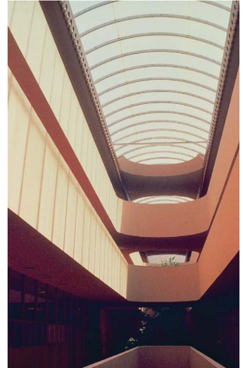
Figure 1.3e In the linear central atrium of the Marin County Civic Center, Frank Lloyd Wright used white surfaces to reflect light down to the lower levels. The offices facing the atrium have all-glass walls.
